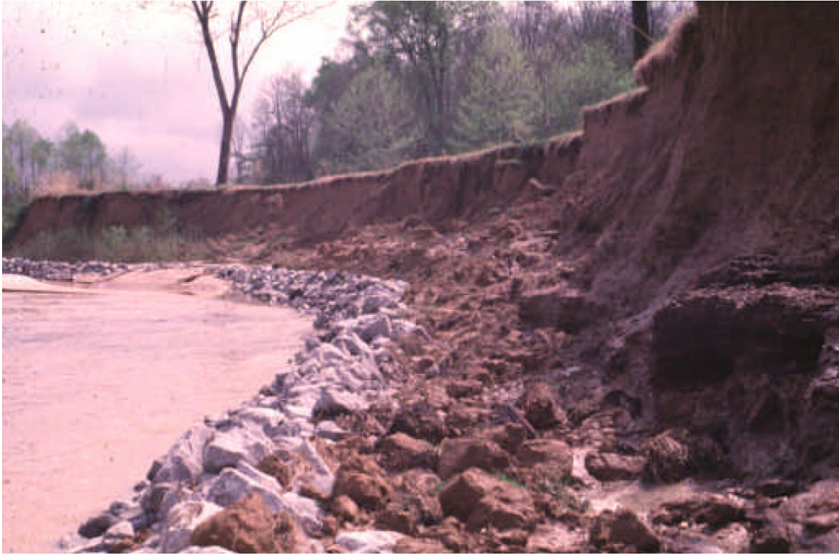
Figure 6-7: Longitudinal Stone Toe - Immediately After Construction (No Bank re-shaping)
