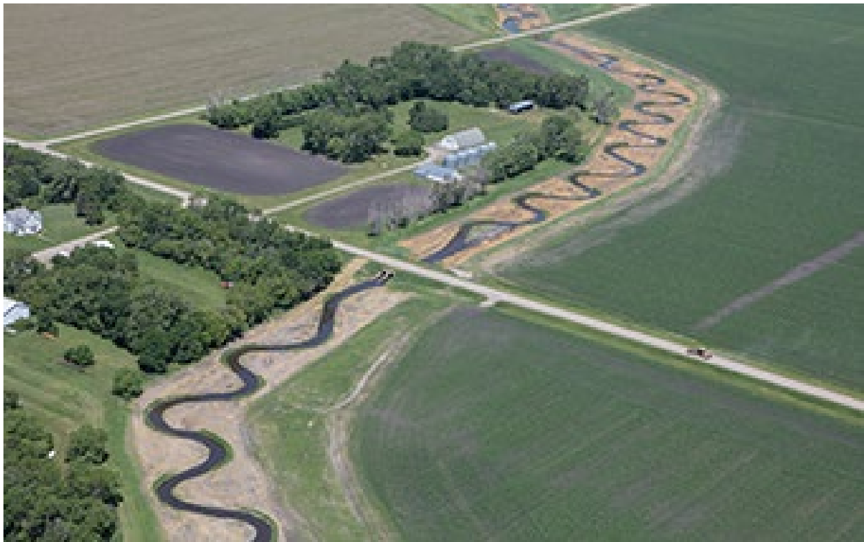
Figure 6-12: Re-meandered Segment of Wolverton Creek (source: Houston Engineering, Inc.)
