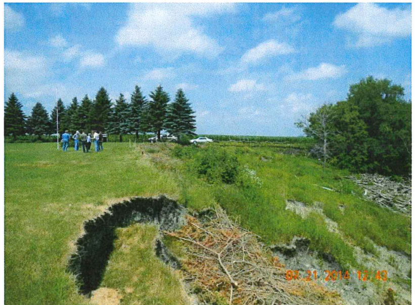
Hemnes Cemetery – Existing riverbank erosion
