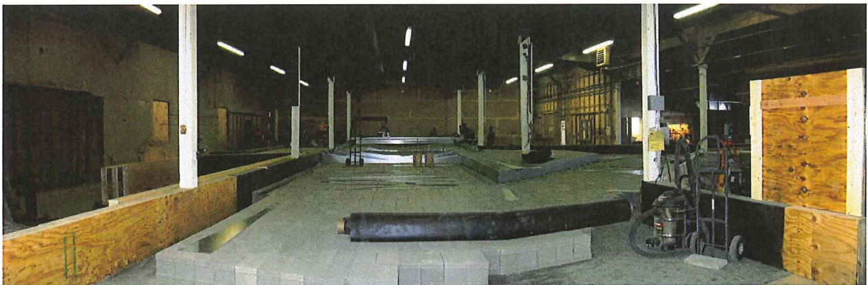
Construction of the Maple River Physical Model
