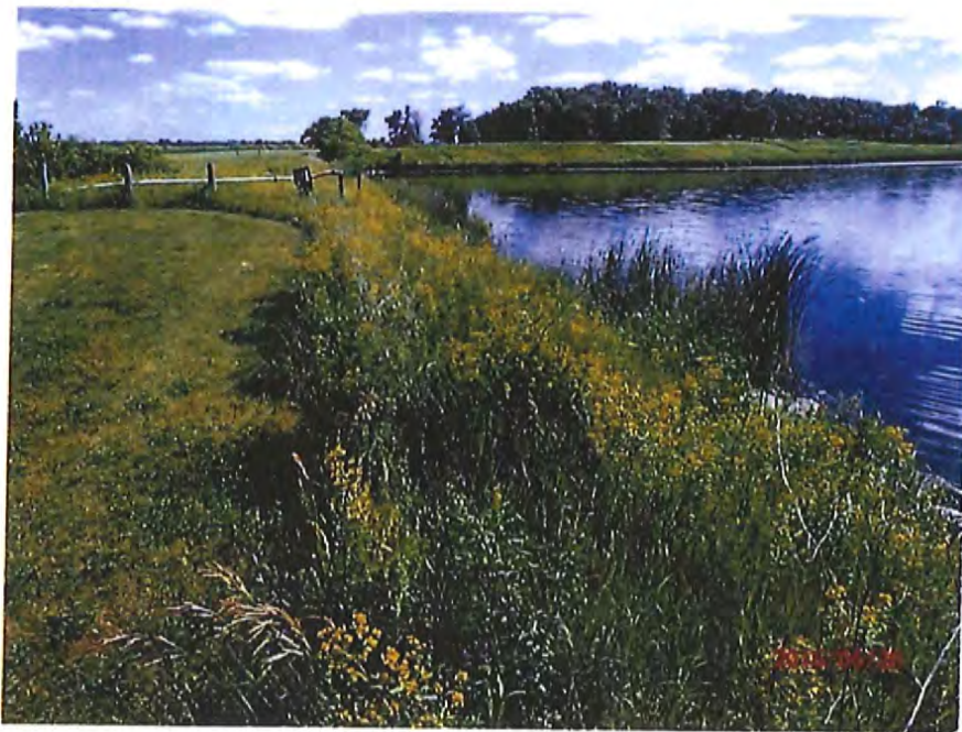
Photo #2 – Upstream slope, looking south.
