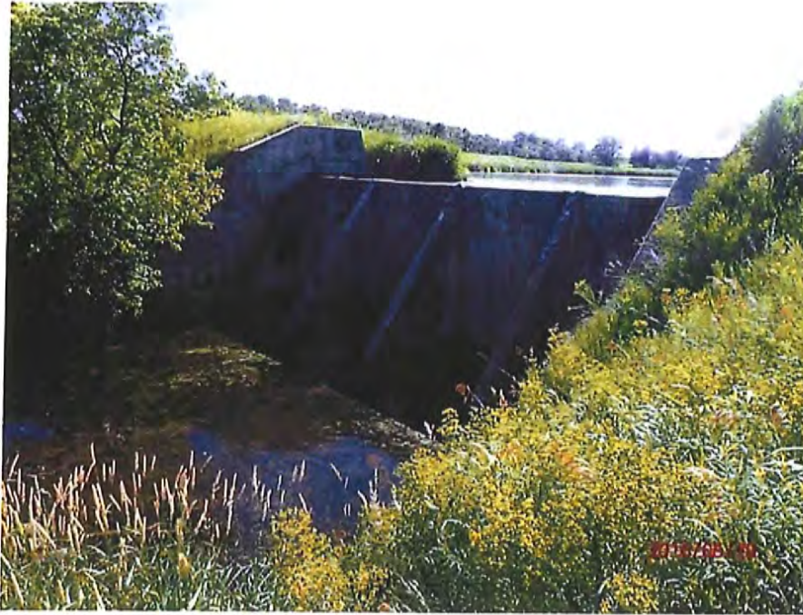
Photo #5 – Principal spillway, looking south.
