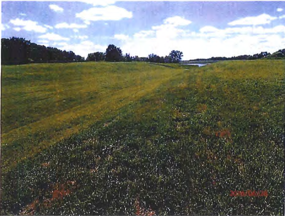
Photo #11 – Emergency spillway, looking upstream.
