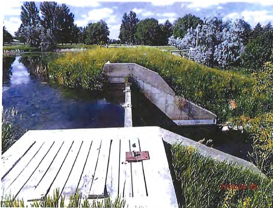
Photo #10 – Principal spillway, looking north. Cover on low level outlet wet well in foreground.
