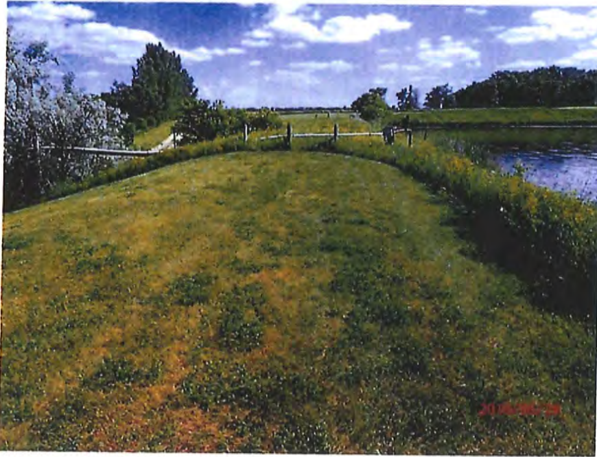
Photo #1 – Hunter Dam, looking south.
