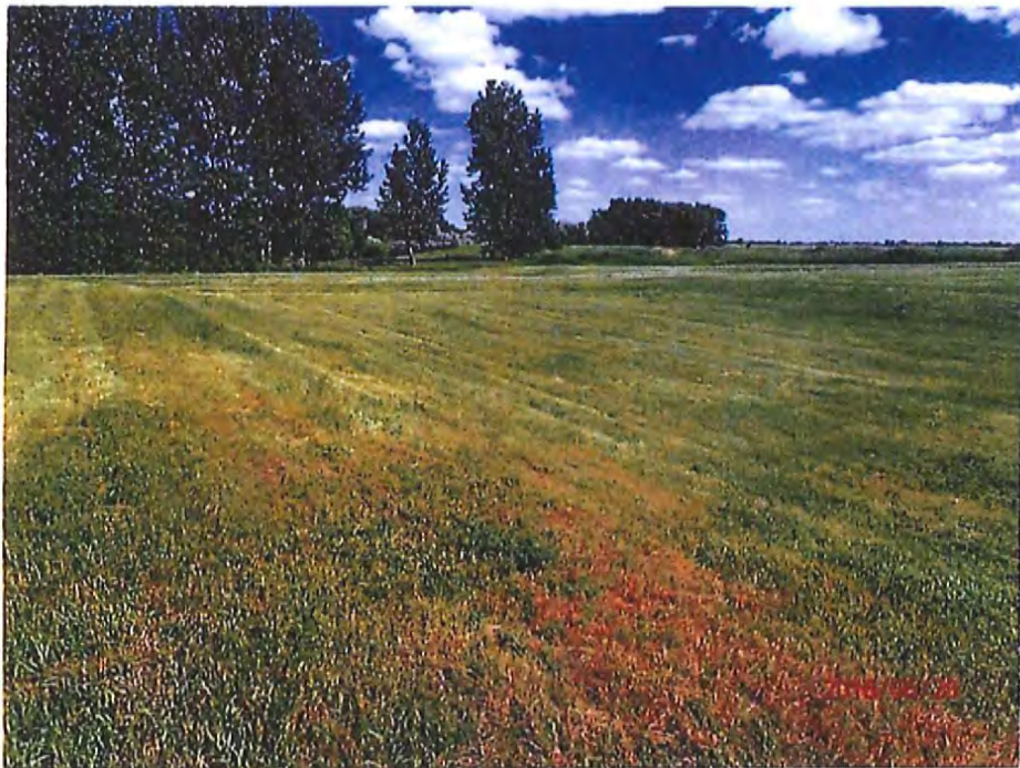
Photo #12 – Emergency spillway, looking downstream.
