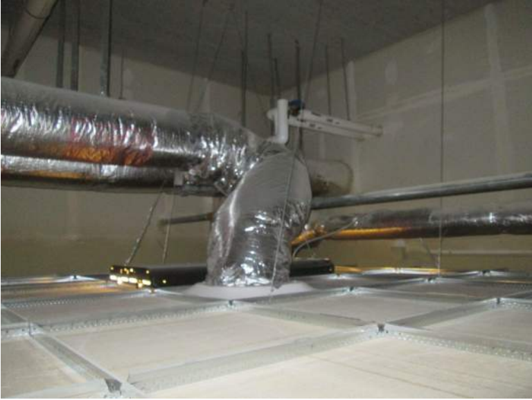
Ceiling space above IT workspace
