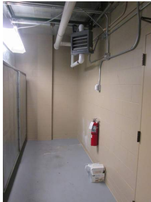
North wall mechanical room @ proposed secure hallway
