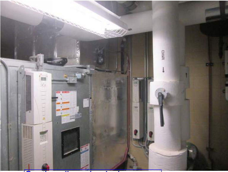
South wall mechanical room
