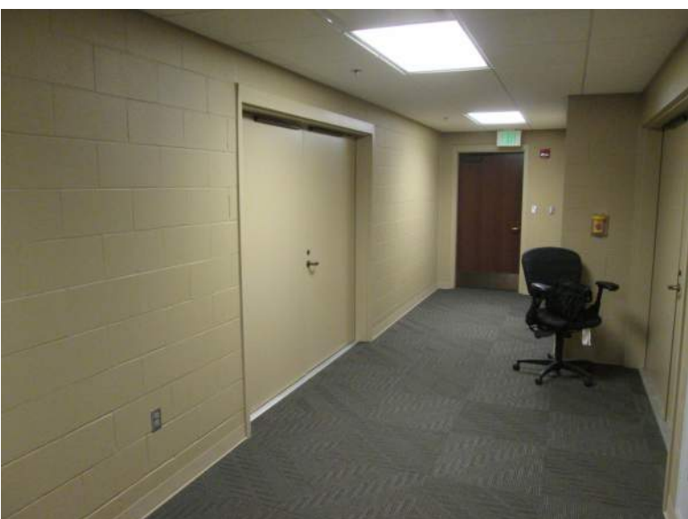
Hallway looking west outside mechanical room
