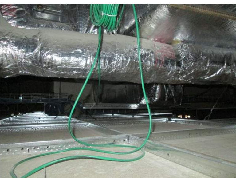
Ceiling space above IT cubicles
