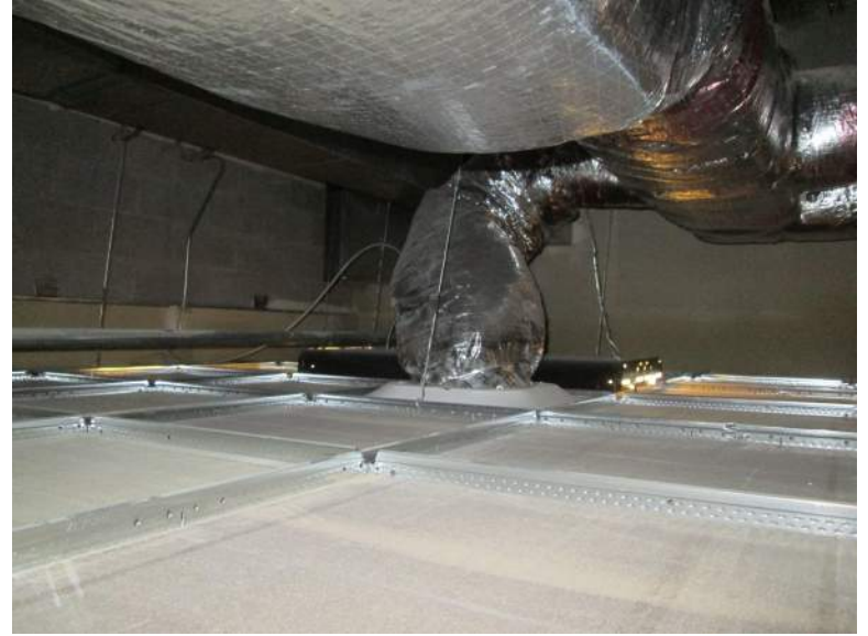
Ceiling space above IT workspace
