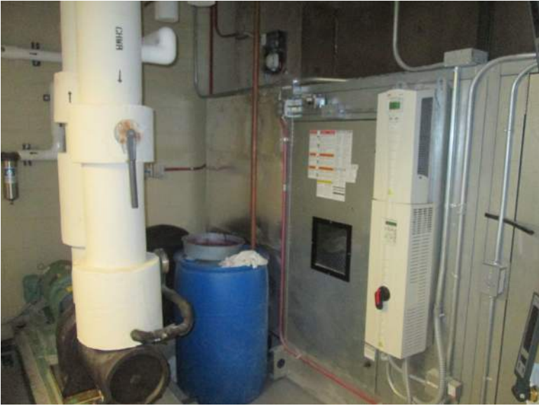
South wall mechanical room
