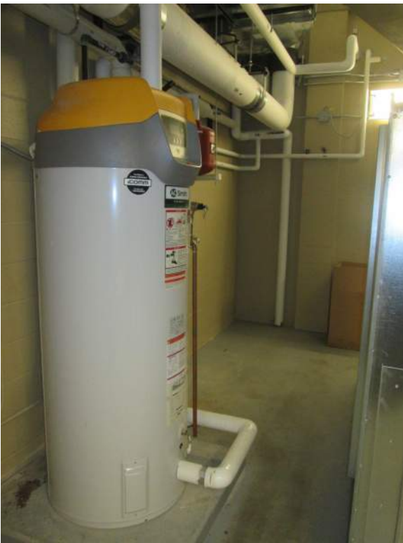
North wall mechanical room @ proposed secure hallway
