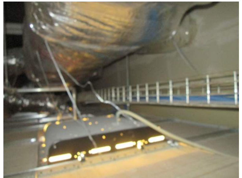
Ceiling space above IT Hallway (N-S)
