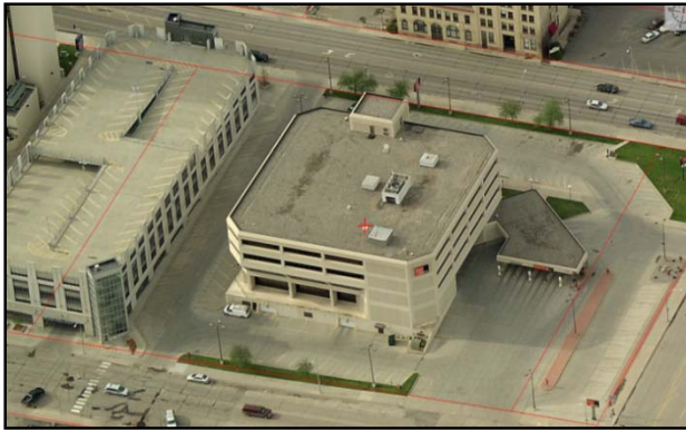
Wells Fargo @ 406 Main Ave – Looking North
