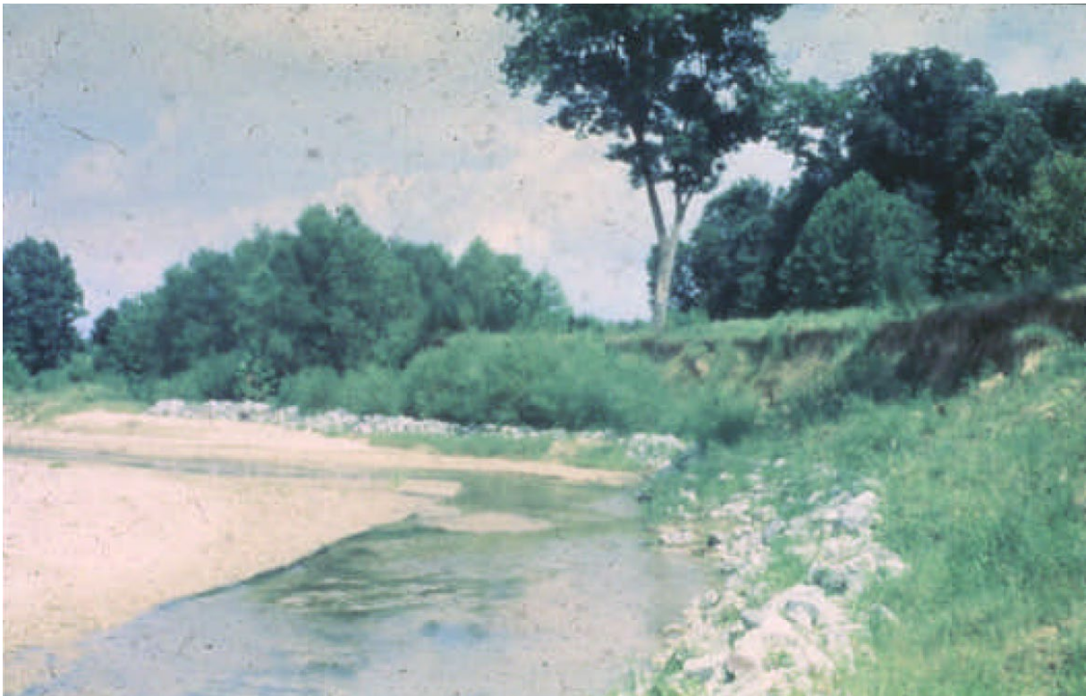
Figure 6-8: Longitudinal Stone Toe – One Year After Construction (No Bank Re-shaping)
