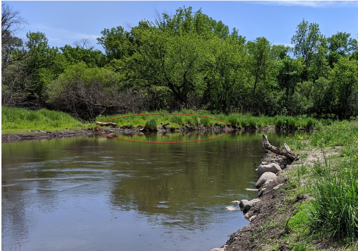
Figure 6-13: Plug of Cut-Off Channel using Toe Wood-Sod Mat on the Pomme de Terre River in Minnesota
