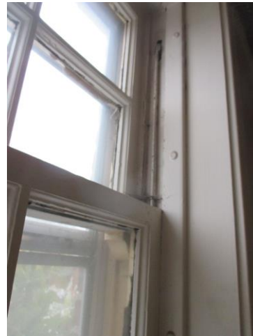
A14: Existing window interior.
