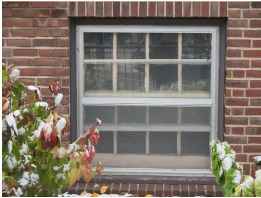
A13: Existing window exterior
