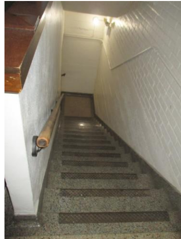
A62: Pyrobar wall block.
