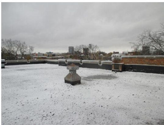
A29: Upper Roof
