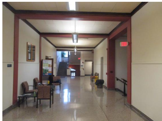
A36: Corridor Finishes
