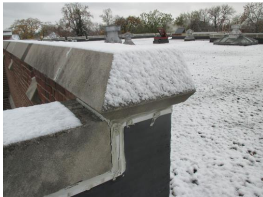
A6: Head joint at window sill
