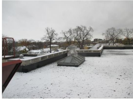
A26: Ballasted Roof.
