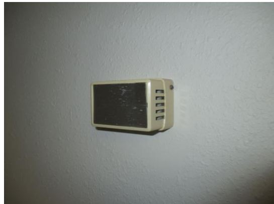
A54: Pneumatic wall control
