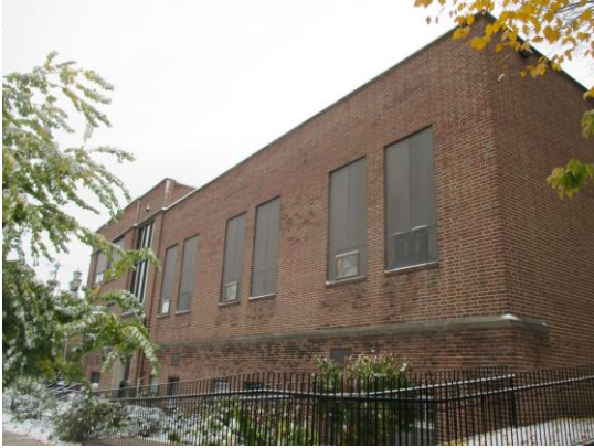
A19: Infilled opening
