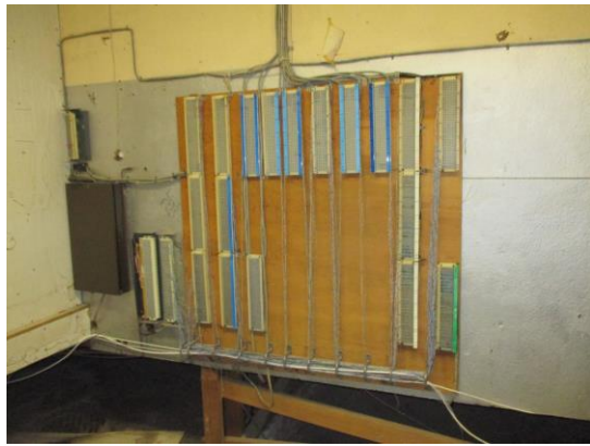
A55: Analog telecommunications panel
