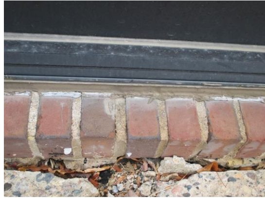
A8: Window sill along grade.
