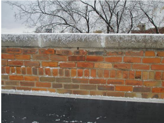
A1: Back of east parapet
