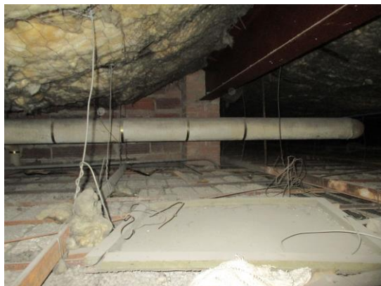
A59: Insulated roof bar joists
