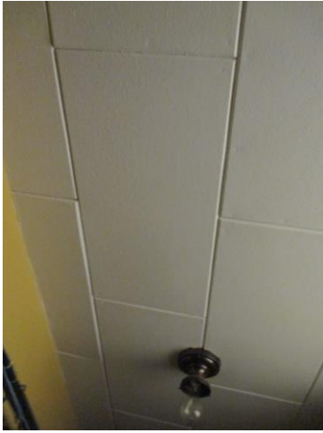
A43: 1x2 adhered ceiling tile
