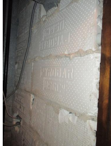
A62: Pyrobar wall block.
