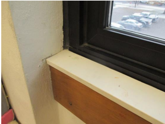
A47: Trim at replaced window
