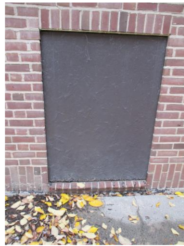
A20: Infilled opening.
