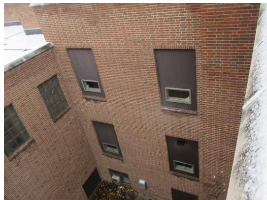
A18: Infilled openings
