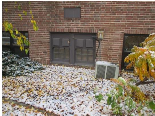
A16: Existing Window Exterior.
