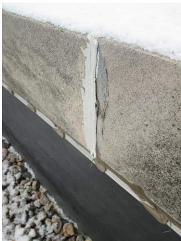
A11: Sealant joint
