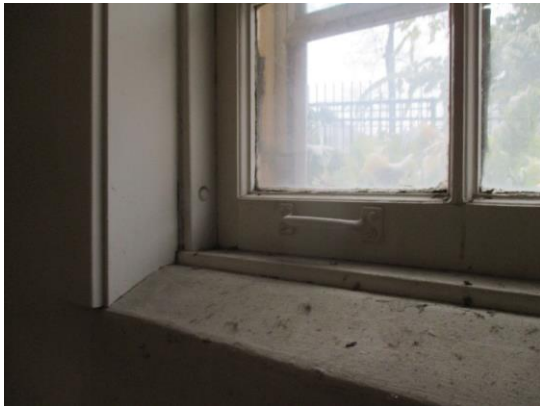
A15: Existing window Interior
