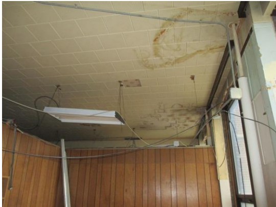
A43: 1x2 adhered ceiling tile
