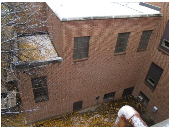
A17: Existing Window Exterior
