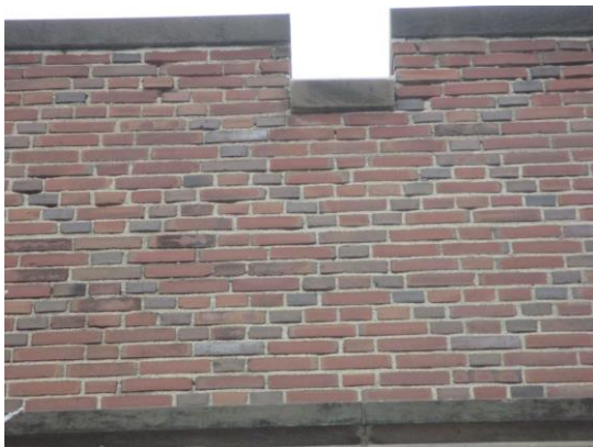
A5: Face of east parapet
