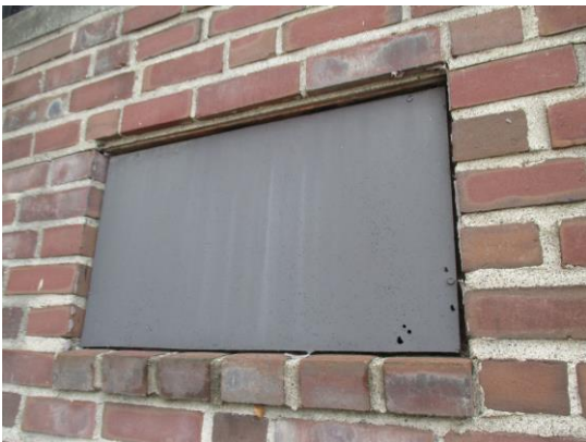
A23: Infilled Opening
