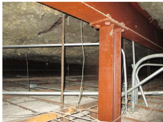
A60: Steel roof support framing
