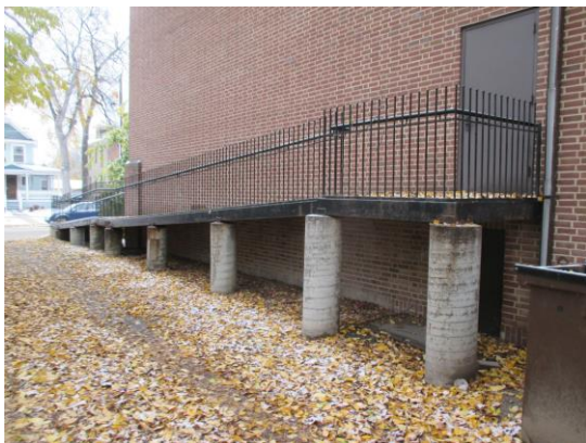
A35: Exterior Ramp
