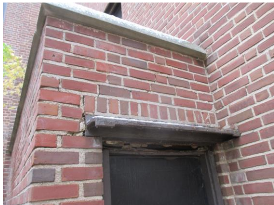
A4: Door head in courtyard.
