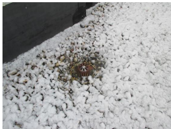
A30: Roof Drain
