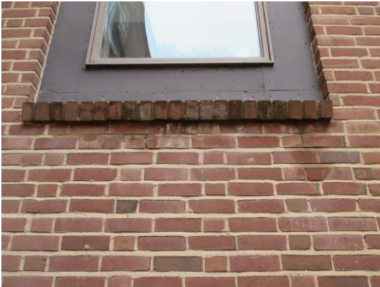
A19: Infilled opening
