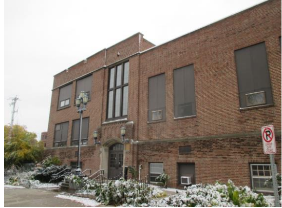
A20: Infilled opening.
