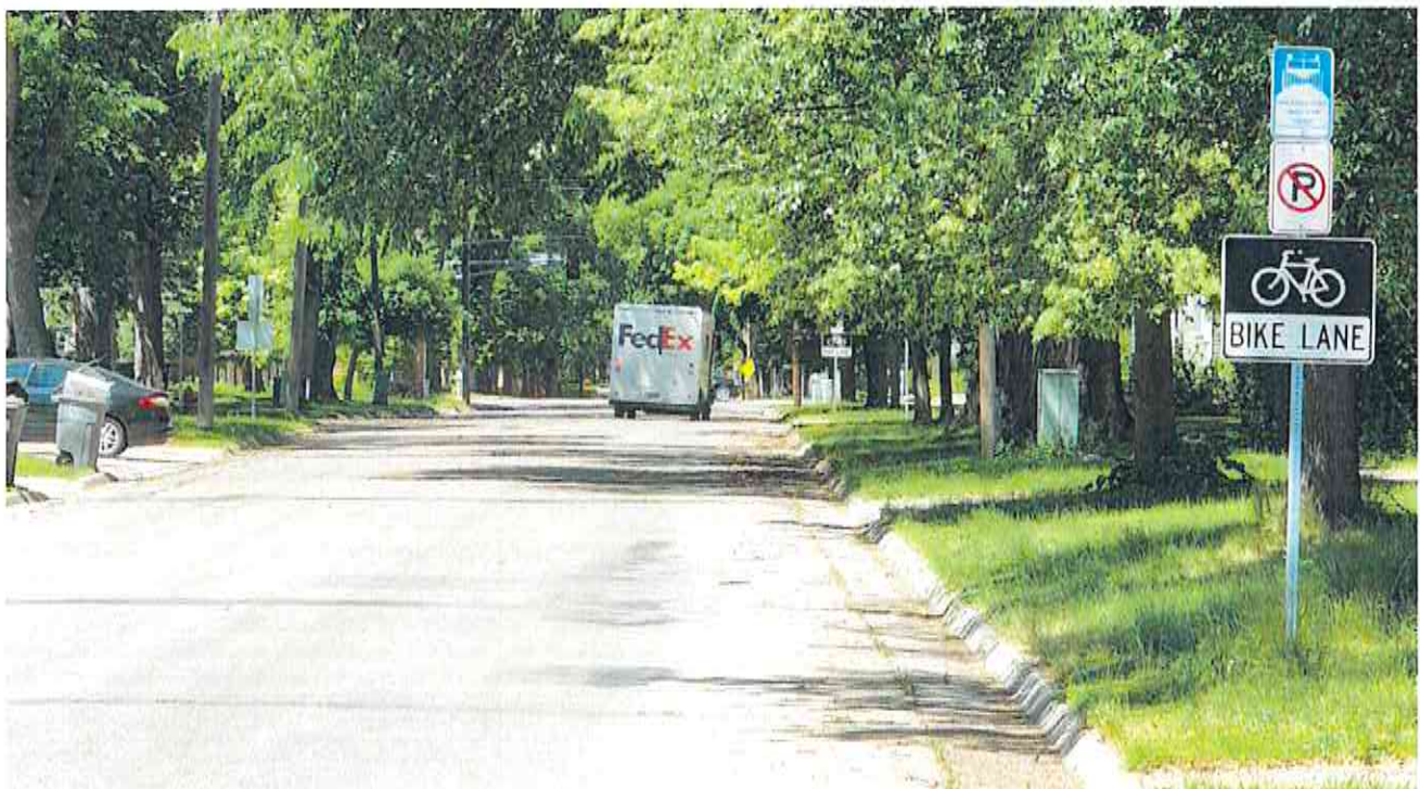
The painted bike lane along 7th Ave in Moorhead is no longer visible; periodic re-application of paint is required to maintain this facility.
