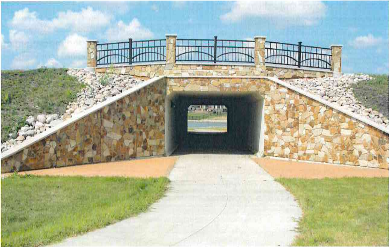
An existing trail underpass in West Fargo
