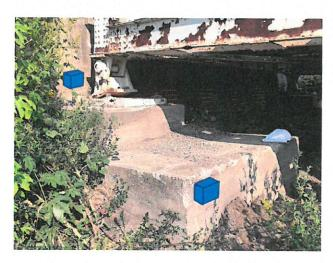
GEOKON has options regarding GeoNet Tilt Loggers, with either integrated Cellular or Radio (wireless mesh) capabilities. Cellular loggers require an additional solar panel for power, while battery-powered Radio loggers require an additional unit (Cellular Gateway) that requires an additional solar panel for power. The various options yield
