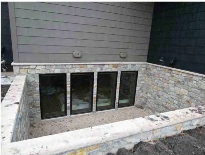
SOUTH SIDE EGRESS WINDOWS
