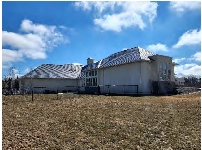
View of the side of the main dwelling
