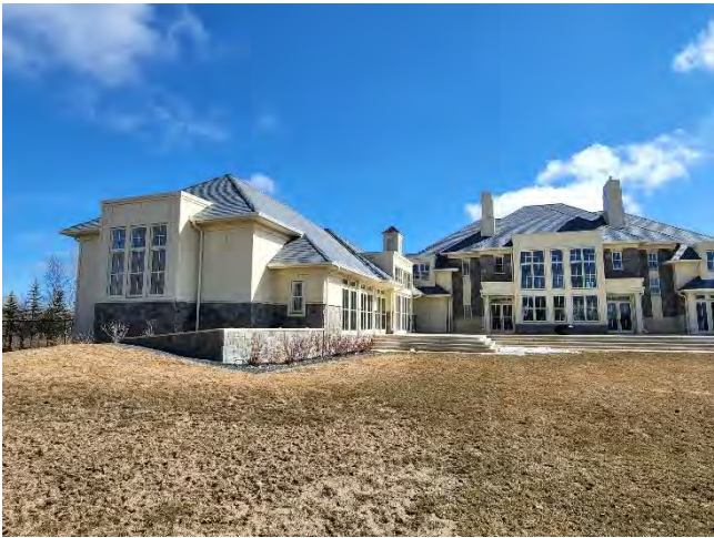
View of the rear of the main dwelling
