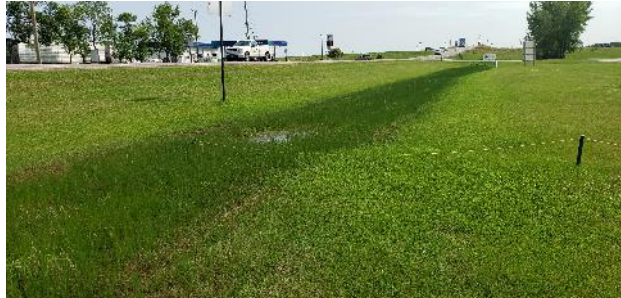
Standing water South of existing Lift Station looking South
