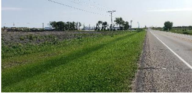
Overhead Power Poles looking south
