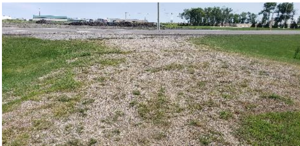
Existing aggregate approach for Lift Station
