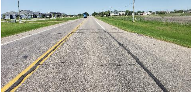
County Highway 11 Roadway Section looking North
