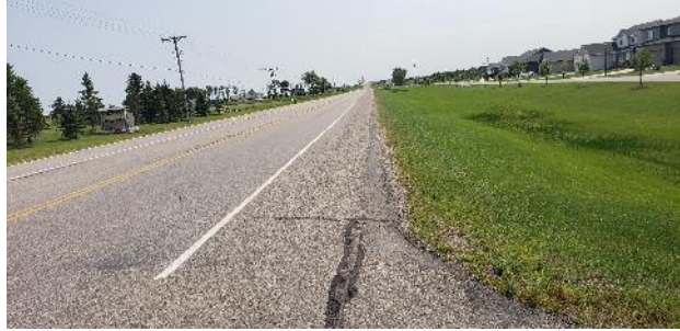
Striped Pedestrian Shoulder looking South
