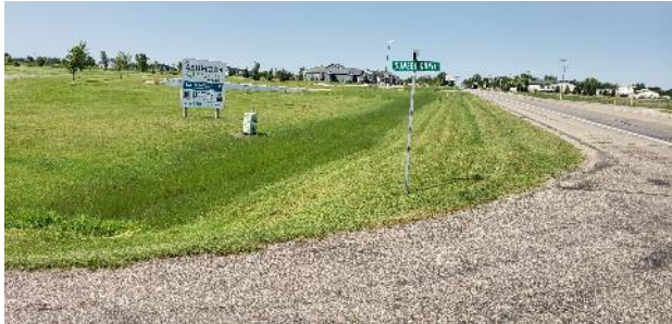
Minimal drainage with soft soils North of Sunset Drive
