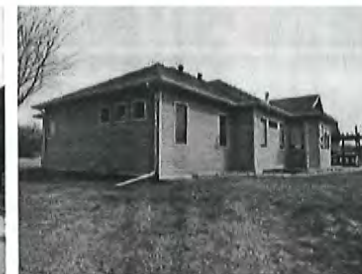
Additional Exterior View
