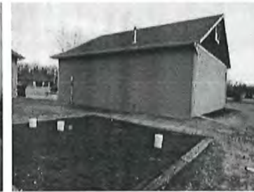
Additional Exterior View
