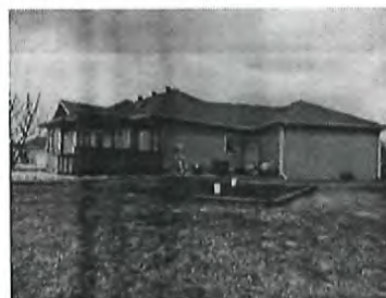
Additional Exterior View
