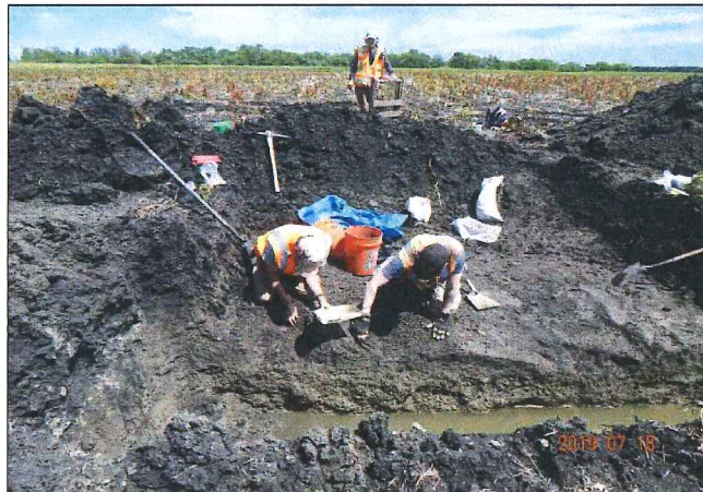
Figure 7. Excavating Bone Cluster in East Wall of Trench 3, Excavated Feature 5 at Left, View East
