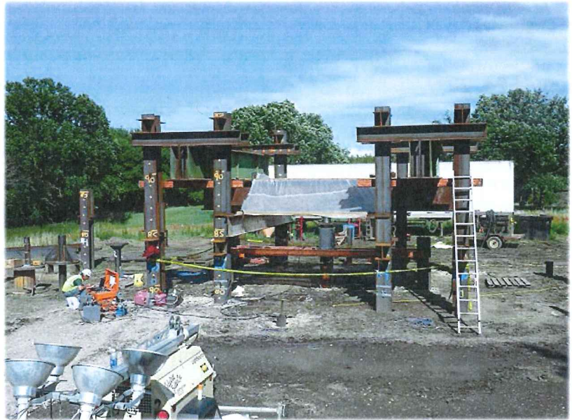
Pile Load Test near Red River – 2012
