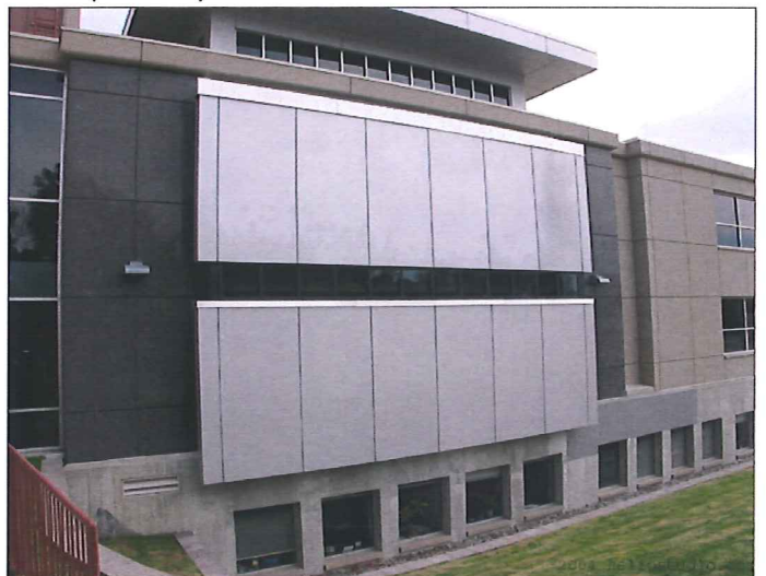
Metal panels were used to screen jury boxes for privacy and security. Natural light penetrates the boxes through the sides of the panels.
