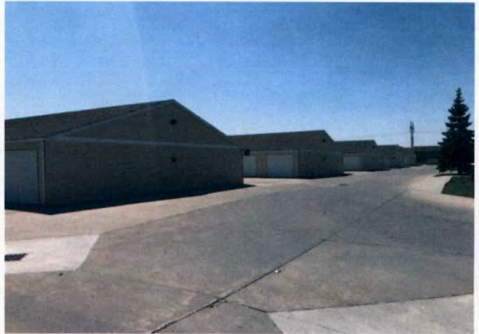
Garage Buildings Looking Southwest
