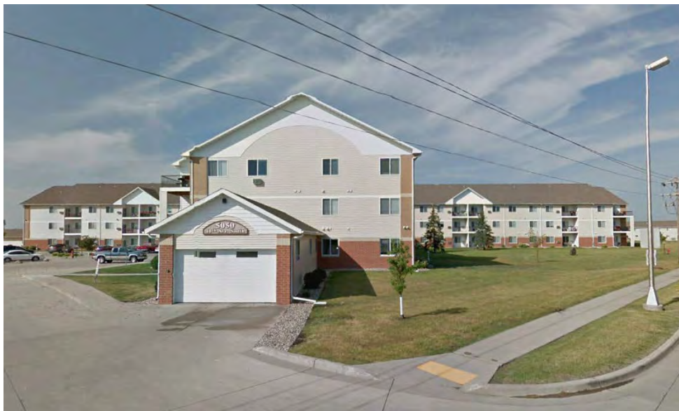
5050 40 Ave S (Looking South from 40 th Ave) Subject Property: Osgood Place Apartments
