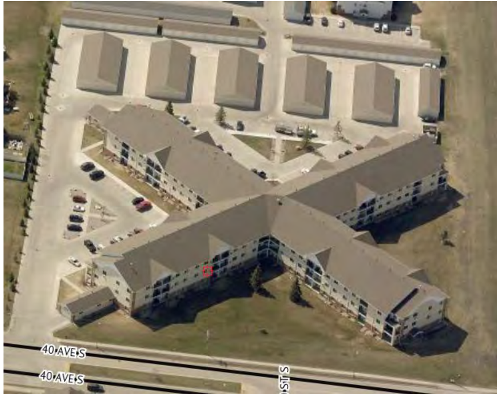
5050 40 Ave S (Looking South) Subject Property: Osgood Place Apartments
