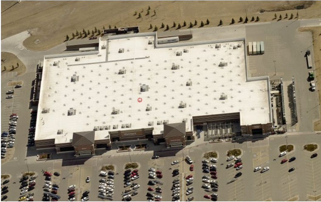
Super Walmart (Front View – Looking East)
