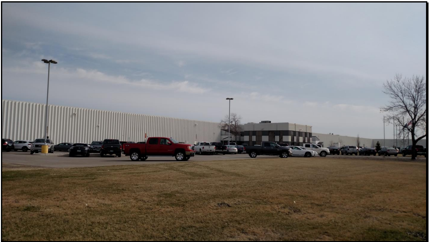
South Elevation View of Main Warehouse
