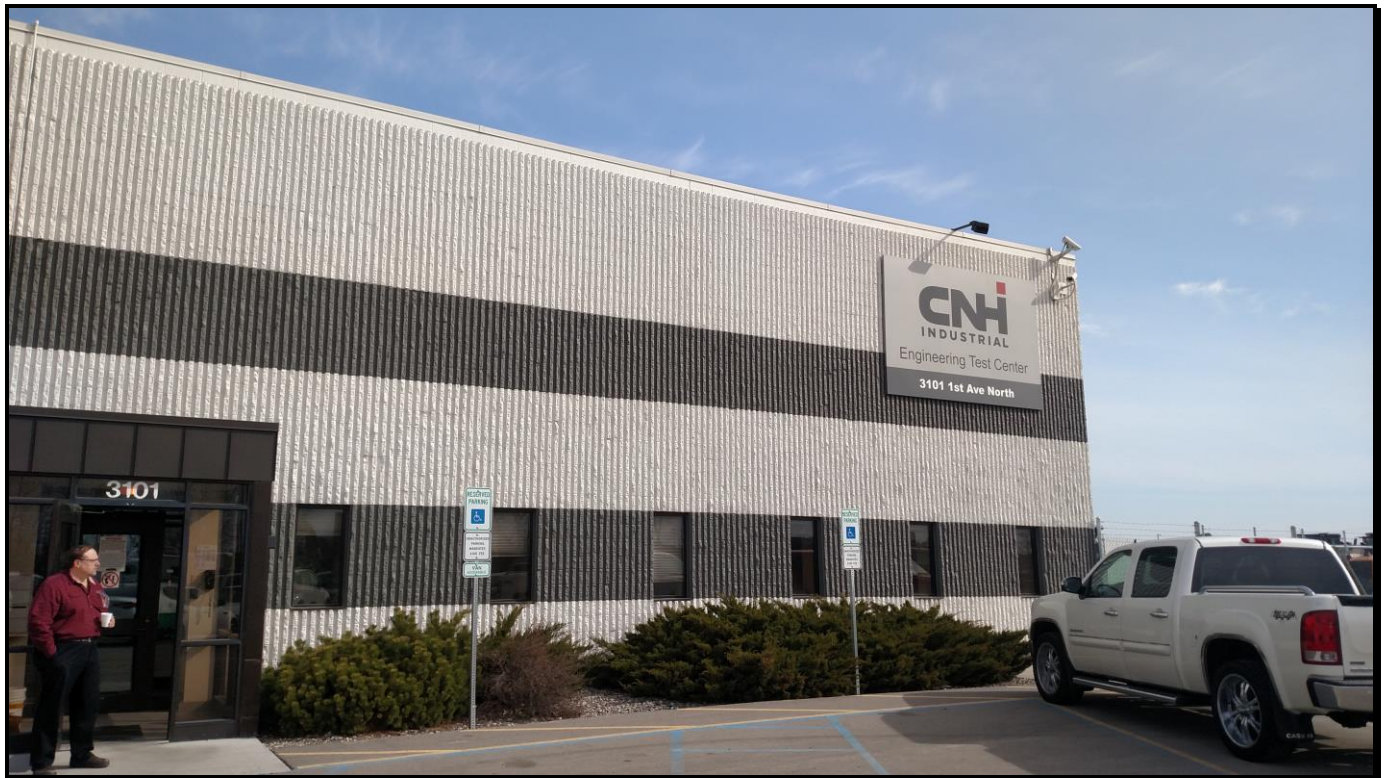
South Elevation View of ETC Building
