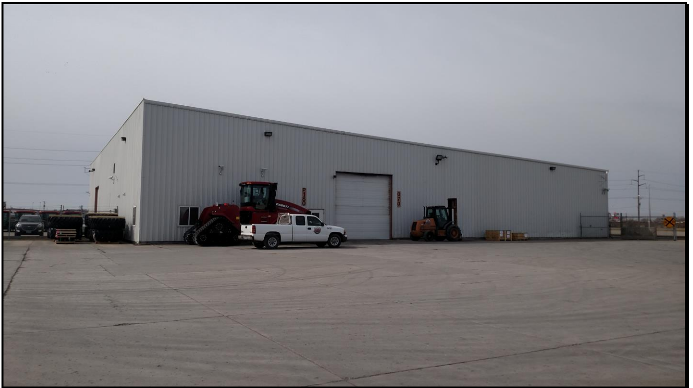
North Elevation View of the Shipping Building
