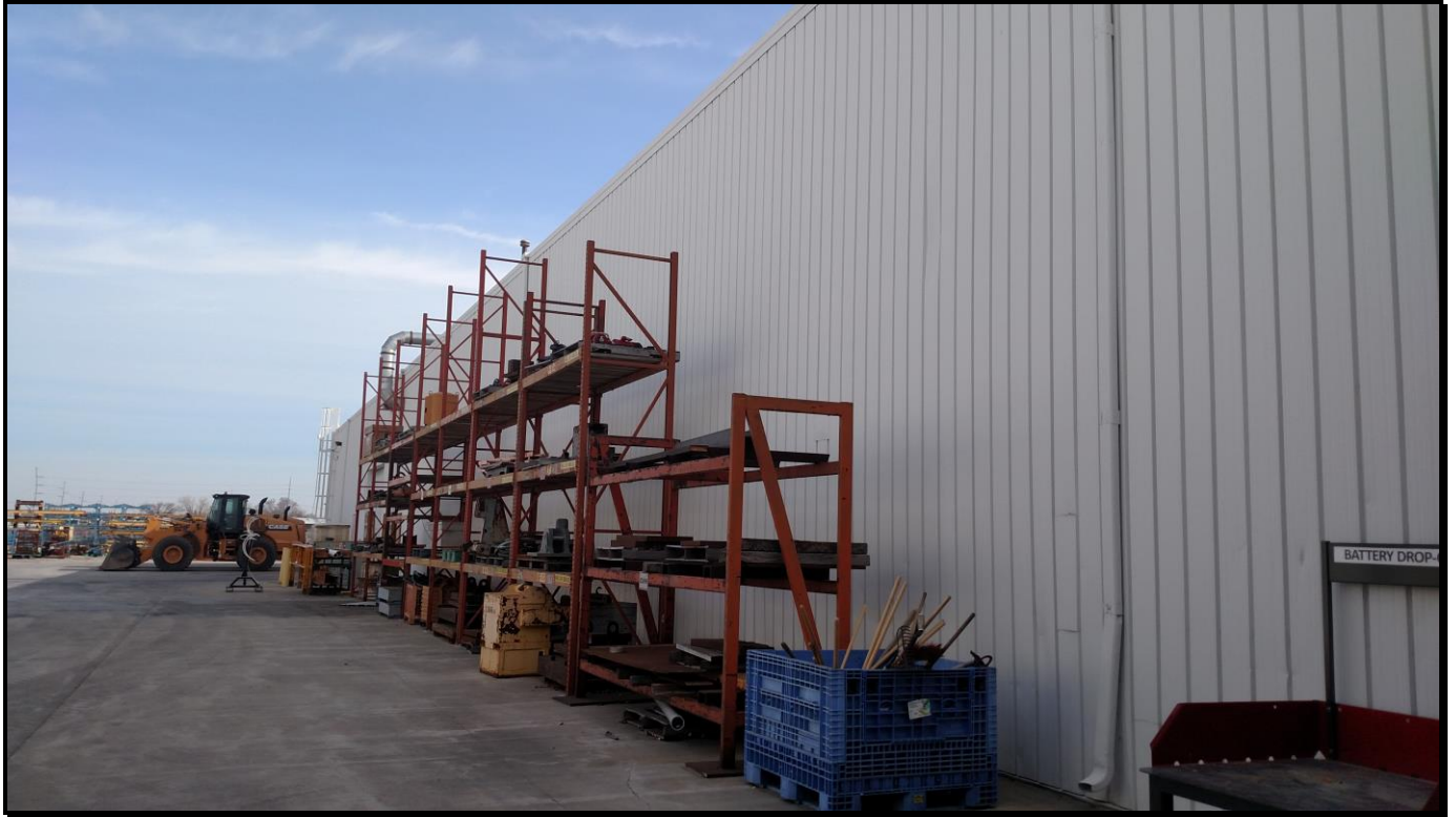
North Elevation View of ETC Building
