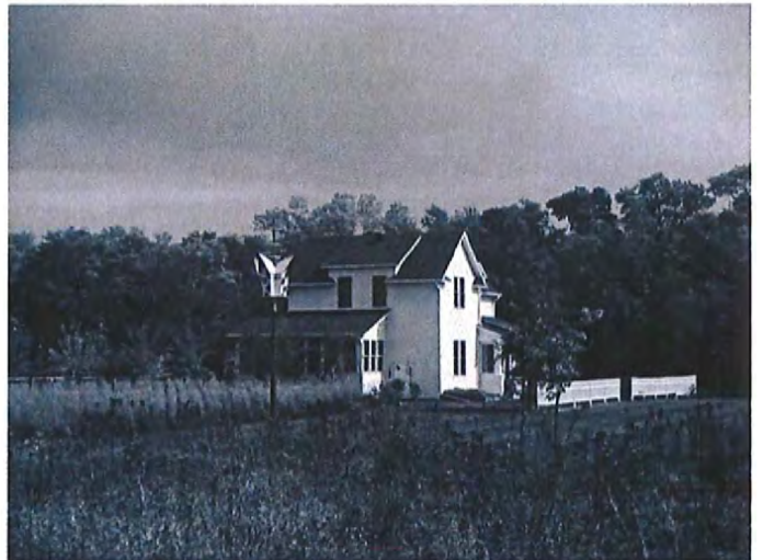
Looking NE towards the Subject Dwelling
