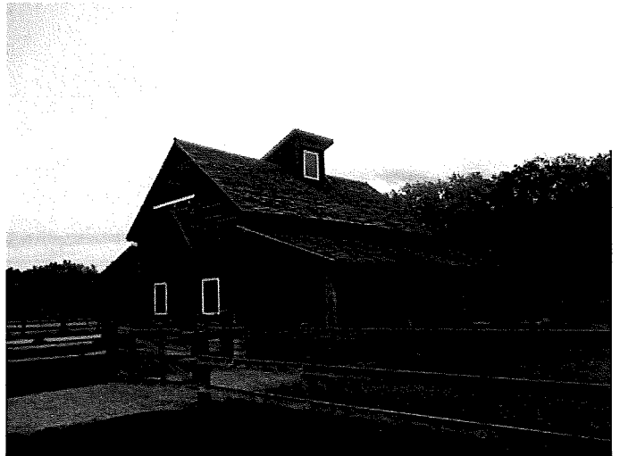
The Stable with Tack Room viewed from the SW looking NE
