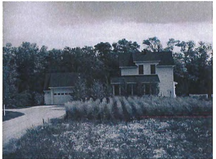
Looking E towards the Subject Dwelling
