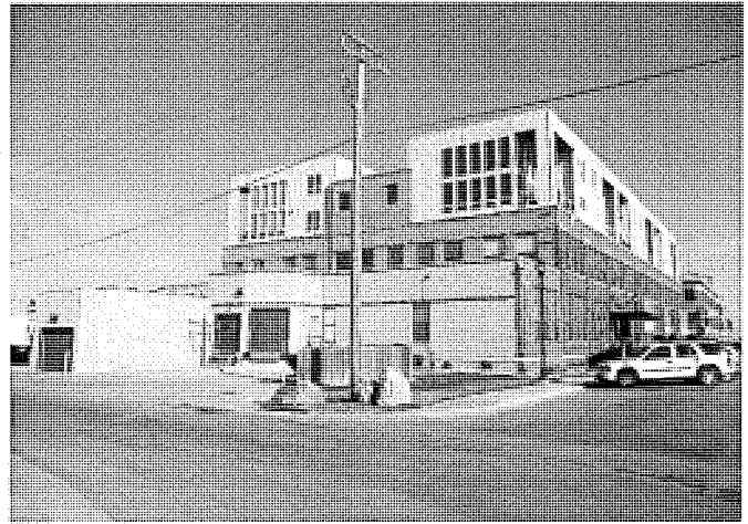
Subject Looking Northwest
